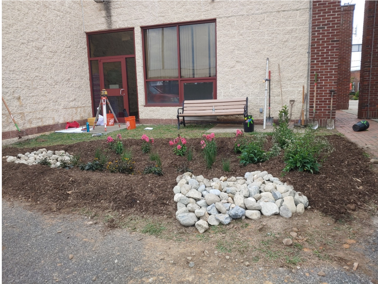
Finished Rain Garden
